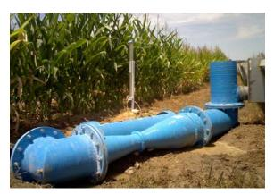
The eQ-pipe 300/125 can be installed in a standardized gate of a prebuilt channel, similar to the Q-pipe 300/125 (discontinued model) shown in the picture, with a gate adapter and 300 mm elbow with reduction (160 mm or 200 mm) where the irrigation hose is connected.
